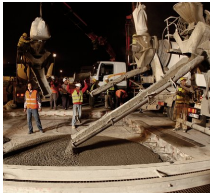
Casting of the new slab
