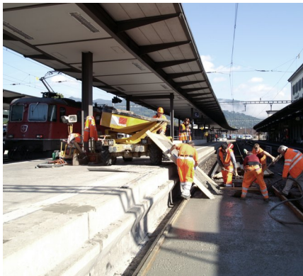
Concrete placement...
