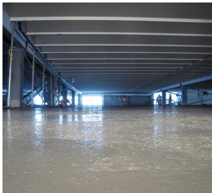
Ground-off concrete surface
