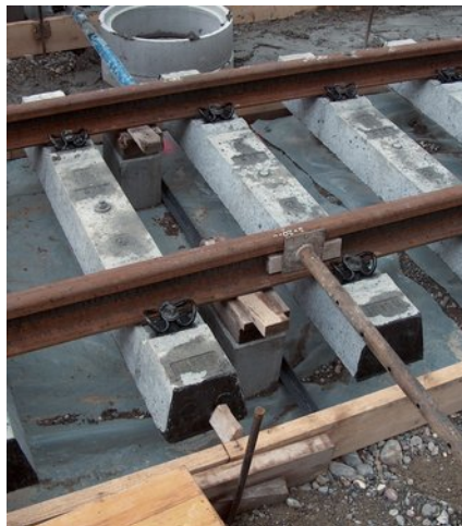
Elevated and aligned track units
