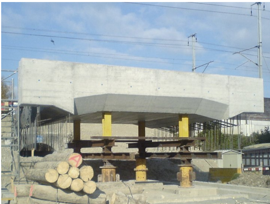
The prepared precast concrete unit before completed with the top plates by ready mix concrete (spaces with visible reinforcing steel)
